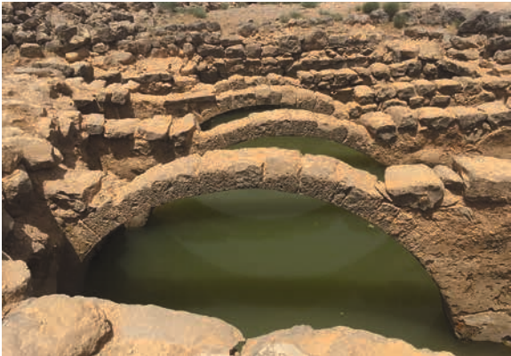
Example of rainwater storage under a house at the archeologic site of Umm al Jimal. Underground, the waters stays clean and cold.
