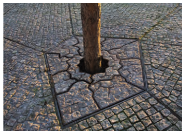
The craquelure pattern of expansion joints and line drains continues into the tree grates
