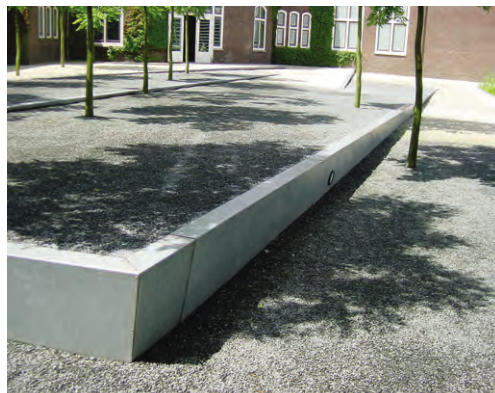
Galvanized steel strips form the edges of the planes. The steel rim leans slightly and as a result the planes seems to float and create a lightness in contrast to the weight of the old building.
